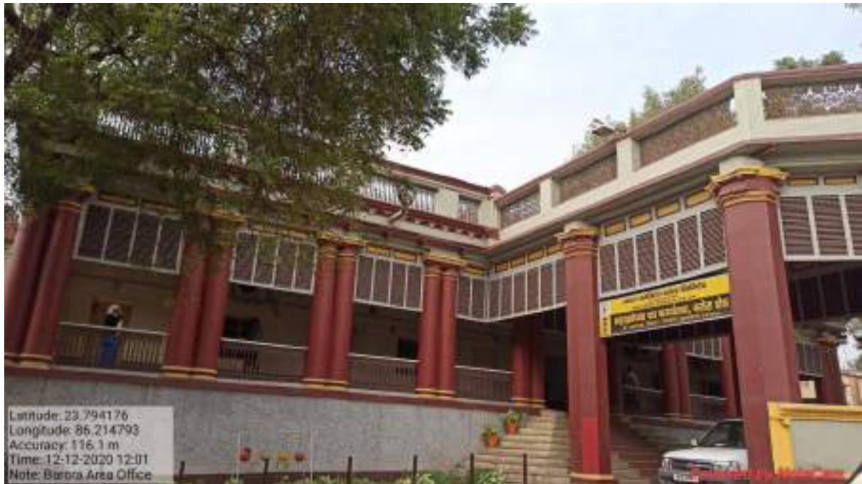
Proposed Rain Water Harvesting Site – Barora Area Office, Cluster-I, Barora Area
